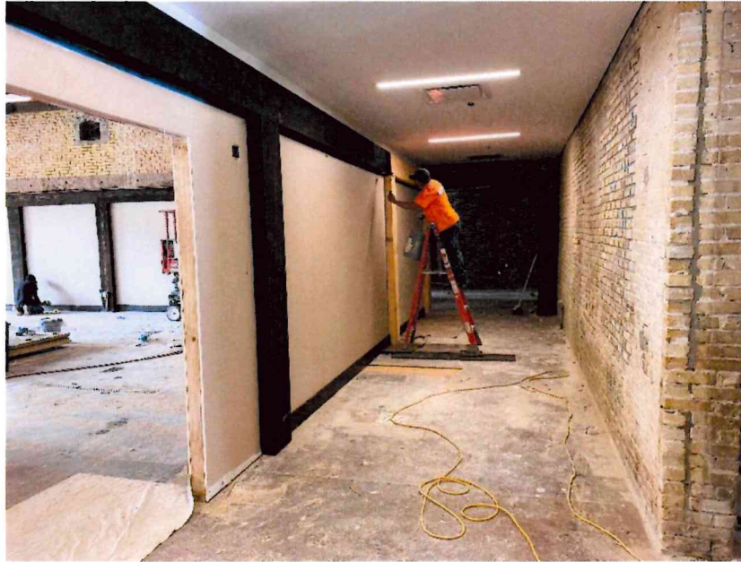
Interior Wood Trim and Stain Installation
