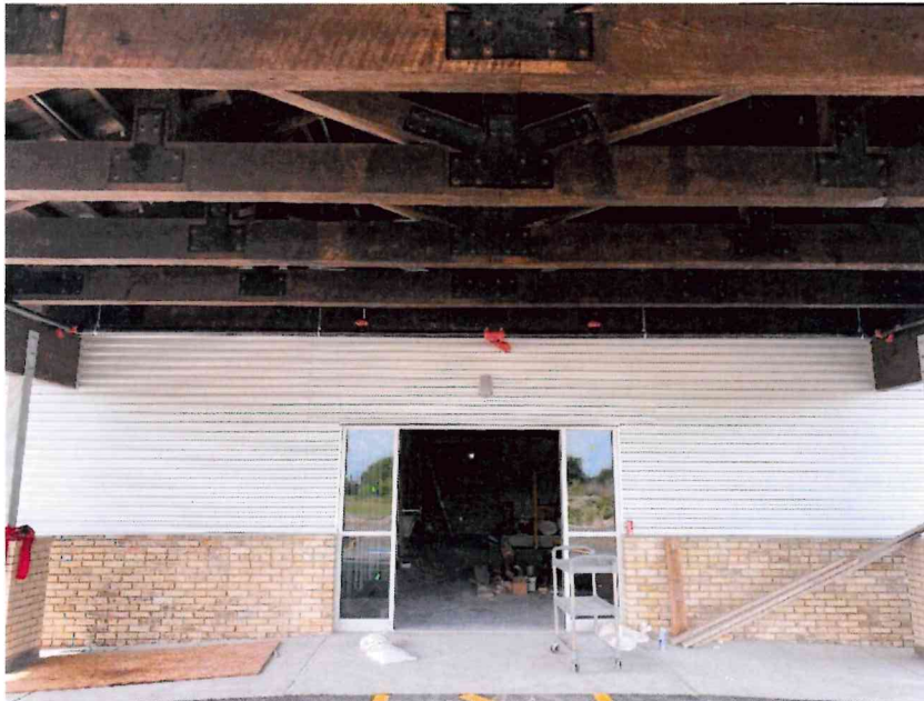
Exterior Aluminum Storefront Installation
