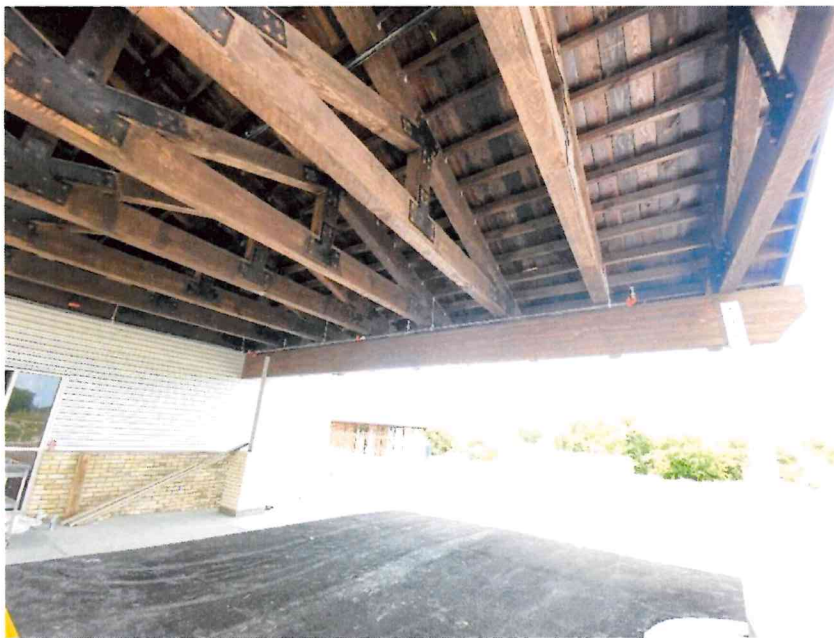
Fire Sprinkler Piping Installation
