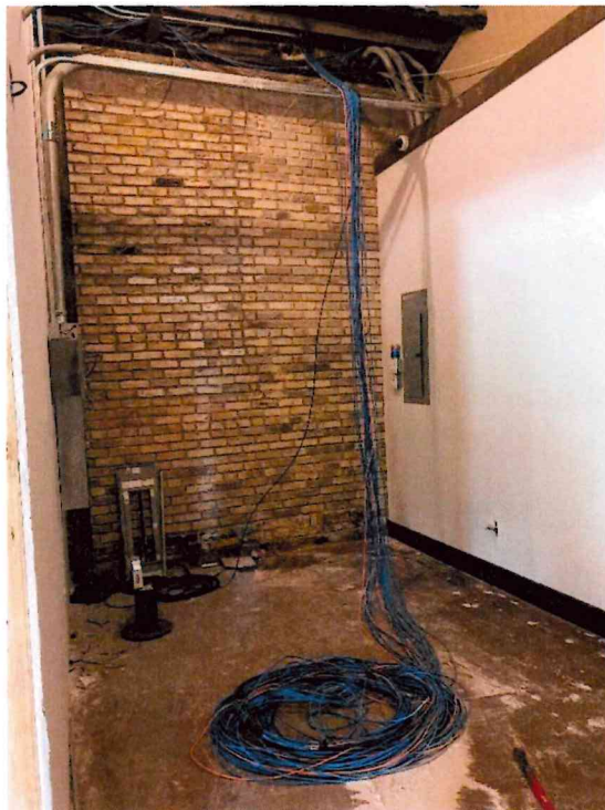
Data Cable Installation
