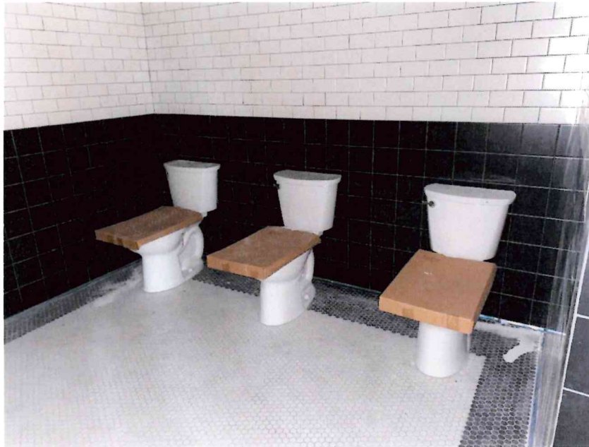
Plumbing Fixture Installation
