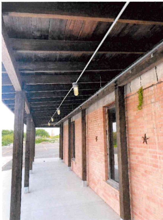
Exterior Canopy Lighting Installation
