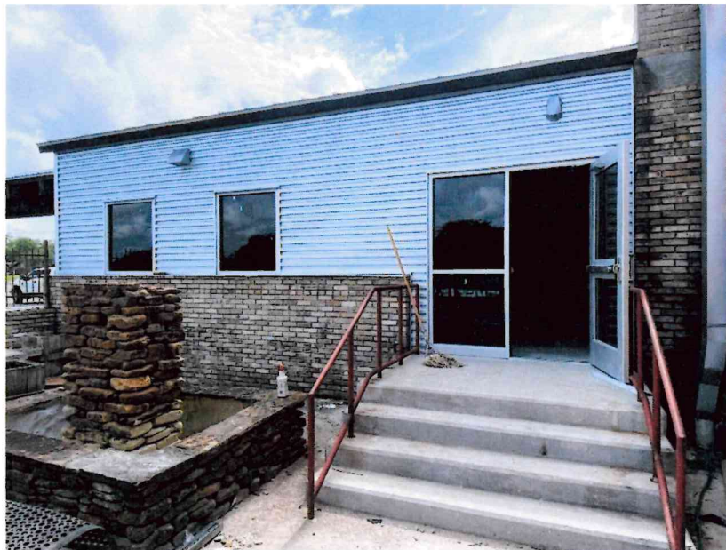
Exterior Aluminum Storefront Installation
