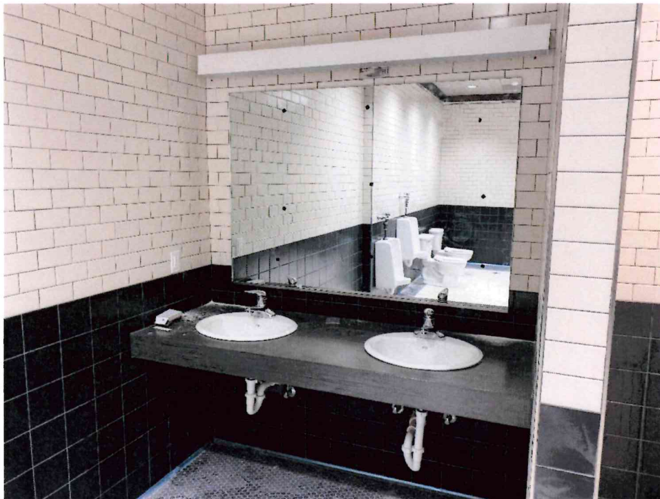
Plumbing Fixture Installation
